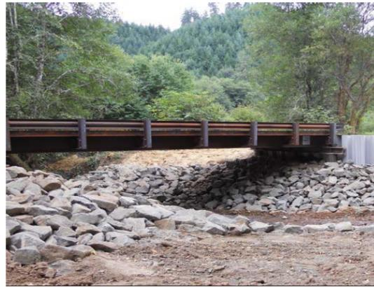
Often culverts are installed for fish passage, but bridges such as this one designed by **Stuntzner Engineering & Forestry** provides fish passage and can sometimes be the right solution for a road crossing.
