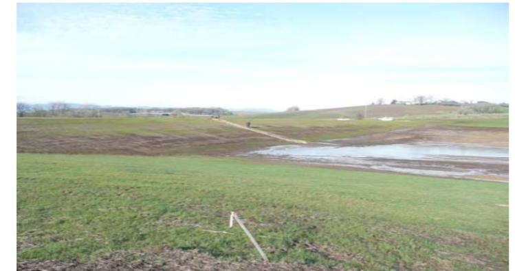
The height of the dam is 27 feet and it has been given a Hazard Rating of "Significant" by Dam Safety. The reservoir, constructed by Eyman Equipment Inc, inundates an area of approximately 12.9 acres and is now approximately 1.7' from being full. Inspections for the initial fill of the reservoir are still on-going. Minor improvements to the dam as well as wetland improvements are proposed for the summer of 2015.
